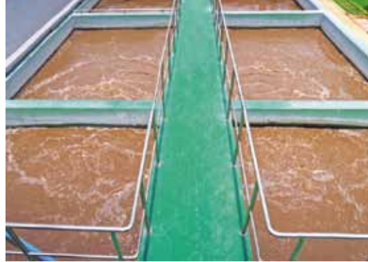
▶ Wastewater treatment: installed at 4.5 meter depth
